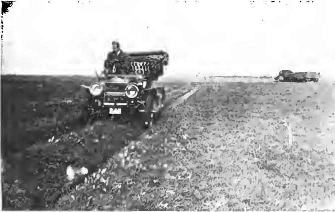
EXPANSE NEAR BETHPAGE SHOWING PARKWAY STAKED.
